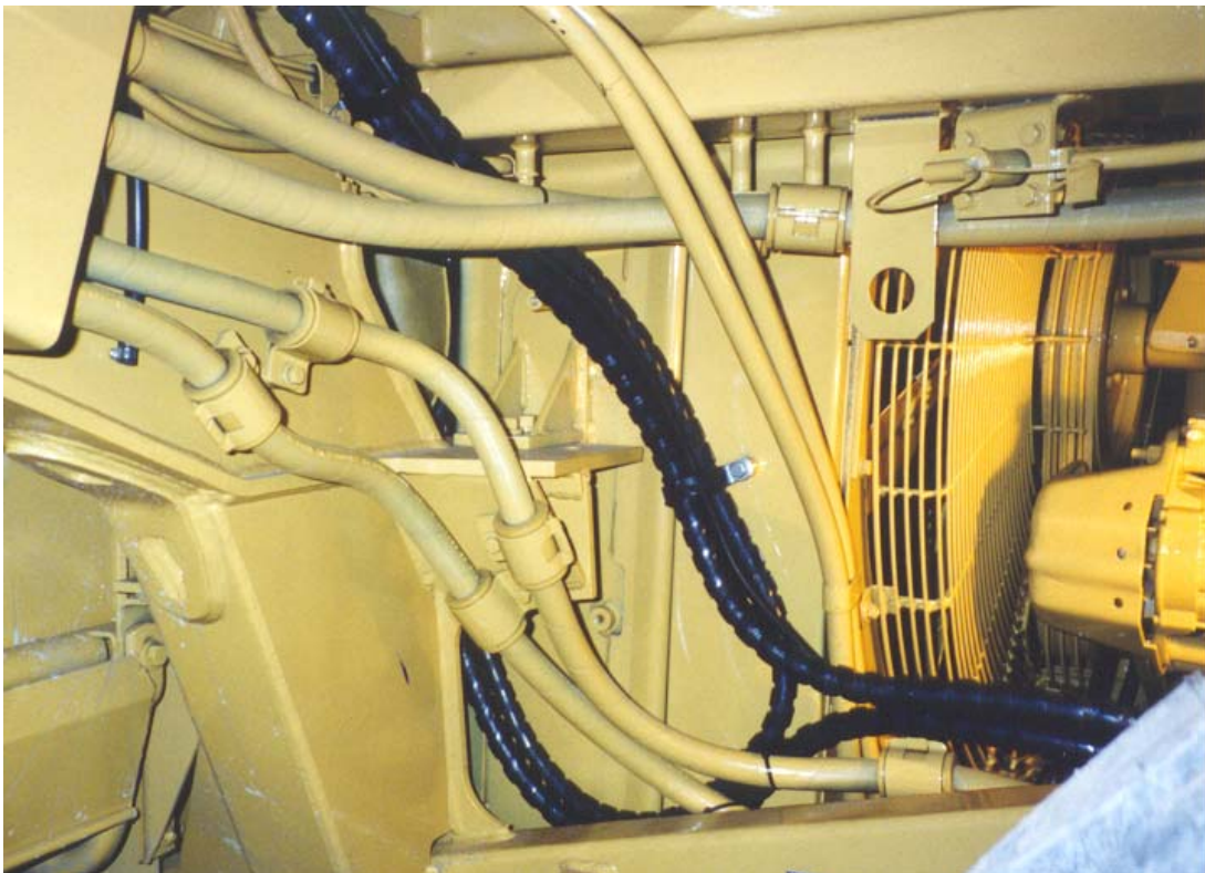
Hose routing in engine compartment of truck.
