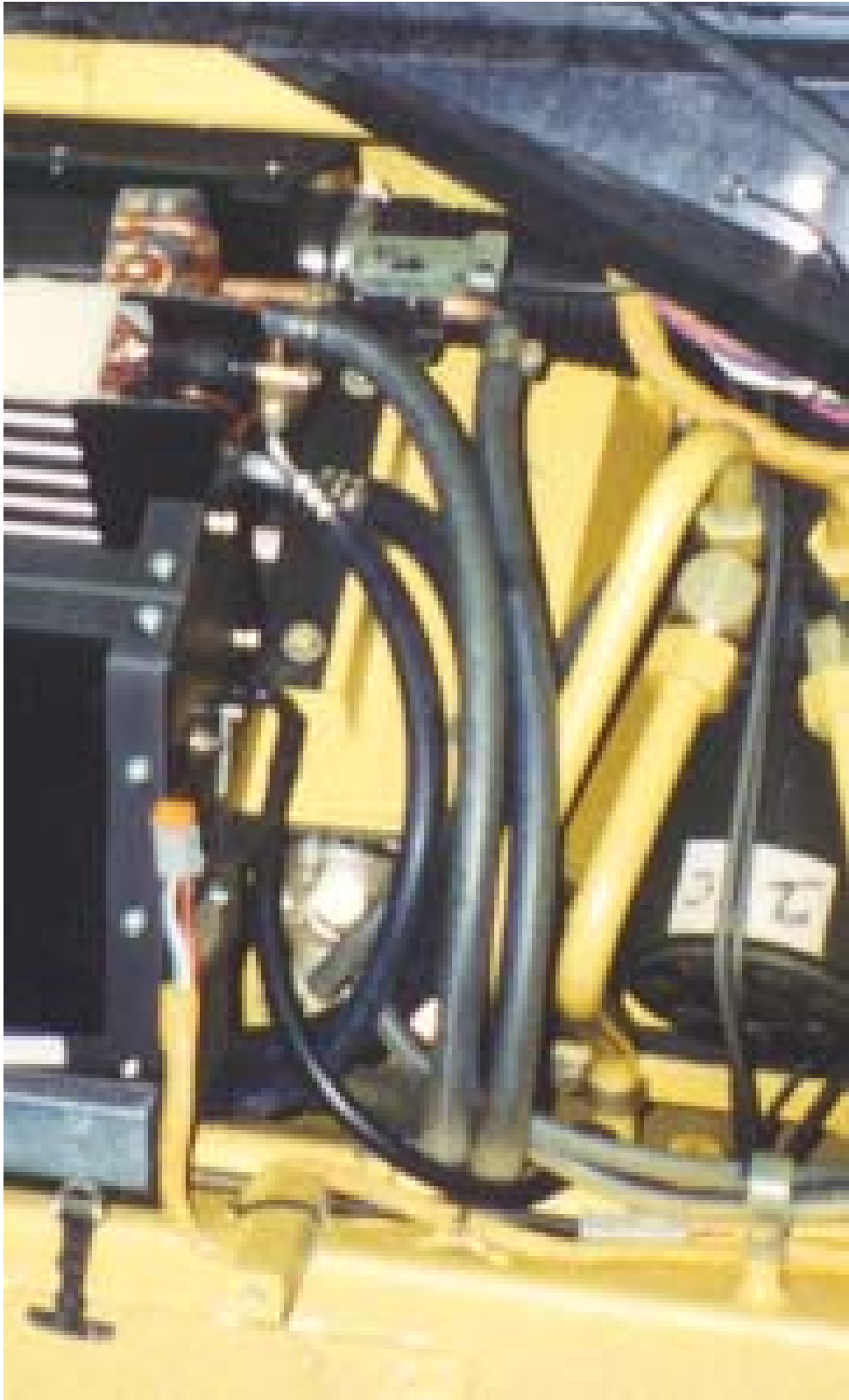
Hoses and routing at evaporator.
