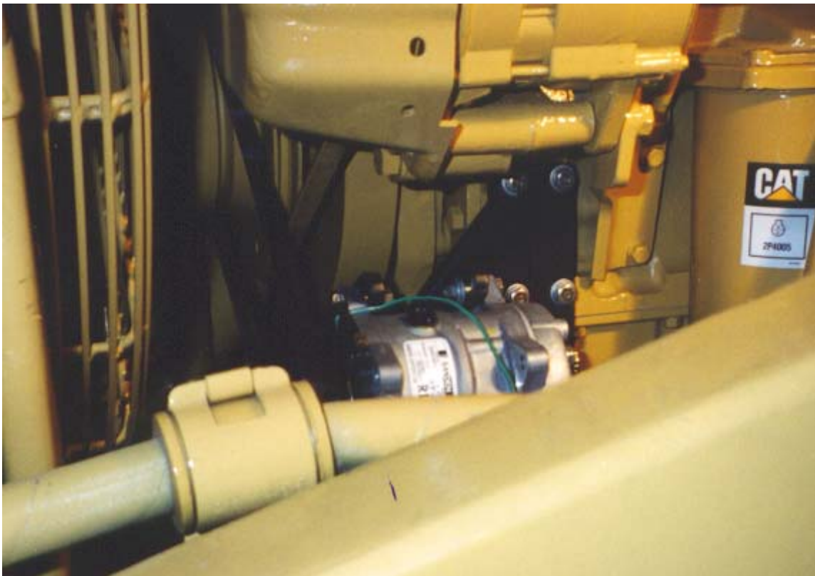
Compressor mounted in place showing bolt locations.
